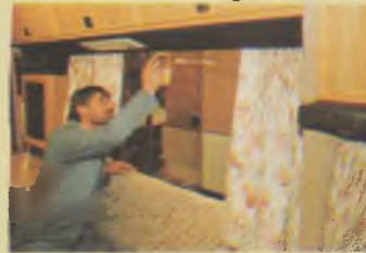
Fitting the lined chintz curtains to runners above the sliding windows.
