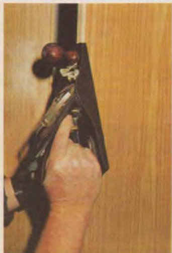
No carefree tolerances here: the hardwood edge of a door is shaved for a perfect fit.
