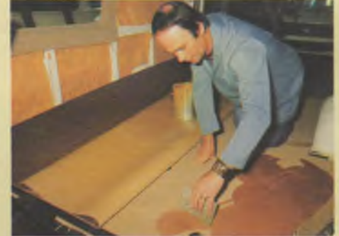
Carpet laying in a Ford Flair. Note the thorough insulation of sidewalls and window surround.
