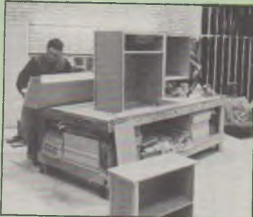
All furniture units are individually prepared prior to installation
