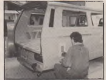
Installing mains electric hook-up prior to fitting of roof and windows
